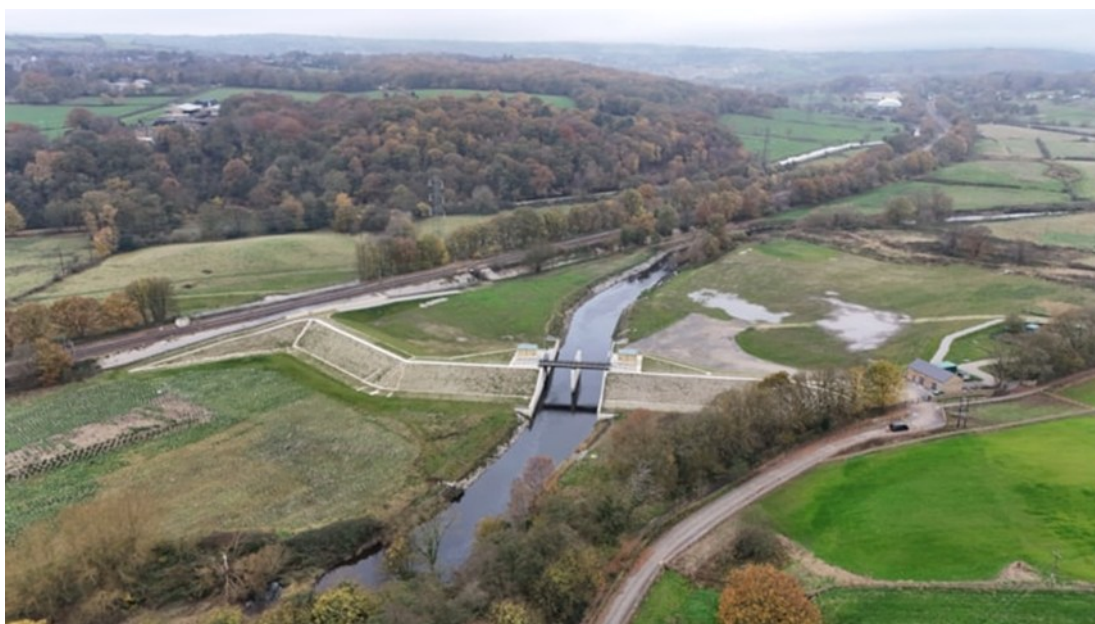
Figure 2 - Aerial shot of temporary flood storage area in Leeds (prior to seeding)
